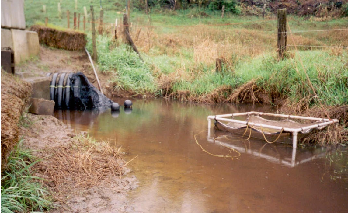
Figure 9. One-way trap at the outflow culvert of the half-round riser water-control structure at Sinko wetland.
